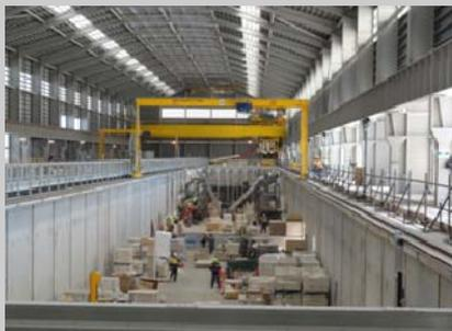
Over 3.5 million refractory bricks were used to line the furnace pits.
